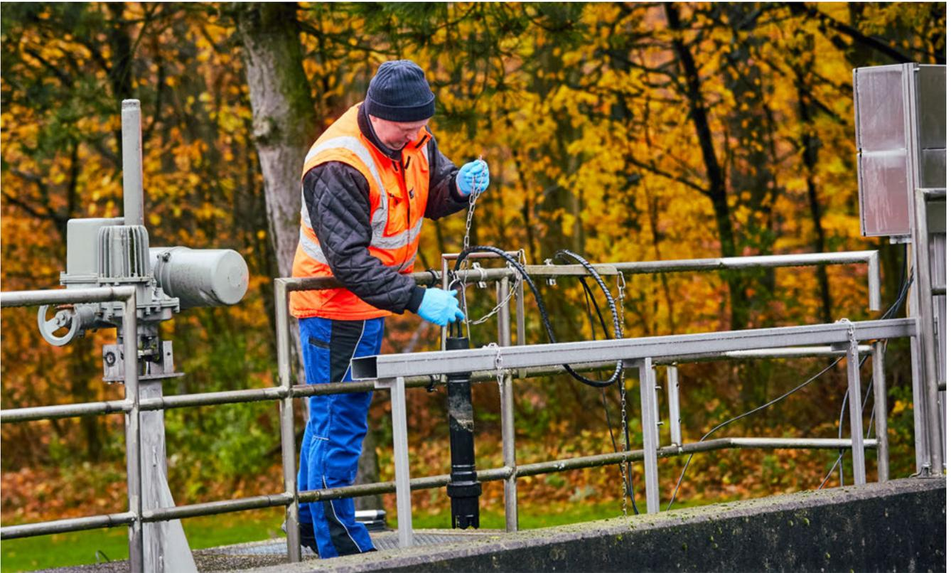
With the ISEmax CAS40D ion-selective sensor, you can measure ammonium and nitrate directly in the aeration basin. This enables nitrogen reduction in the biological phase to be controlled based on load – and the process to be optimized.
