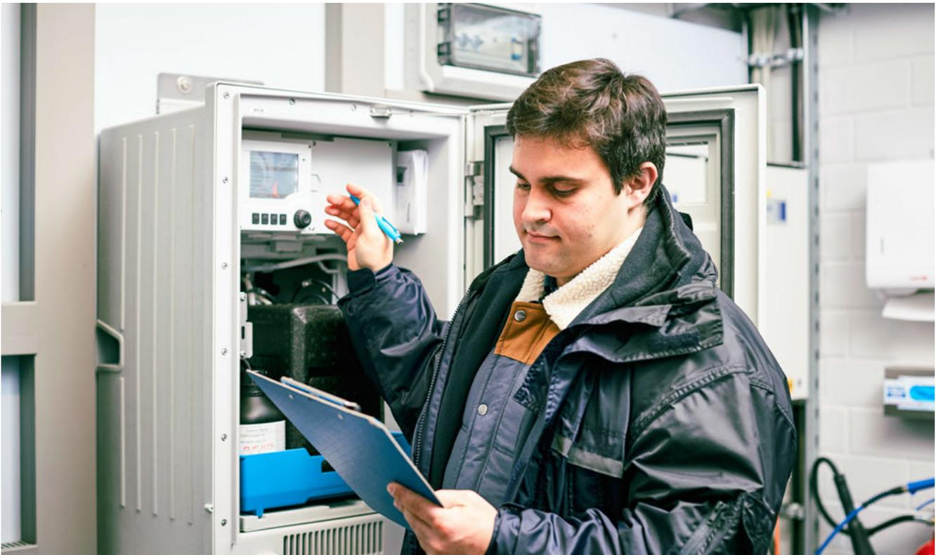
The orthophosphate analyzer, Liquline System CA80PH, provides reproducible measured values for reliable precipitant dosage.
